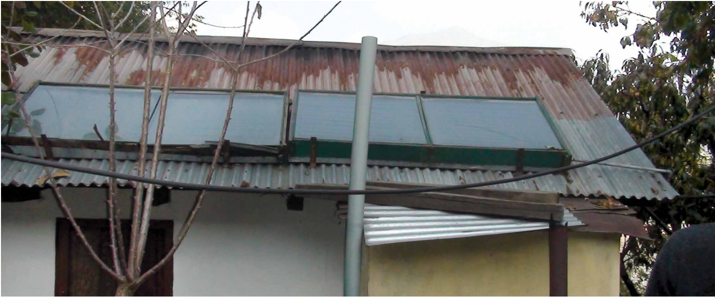
Leelawati's house with solar water heating system
