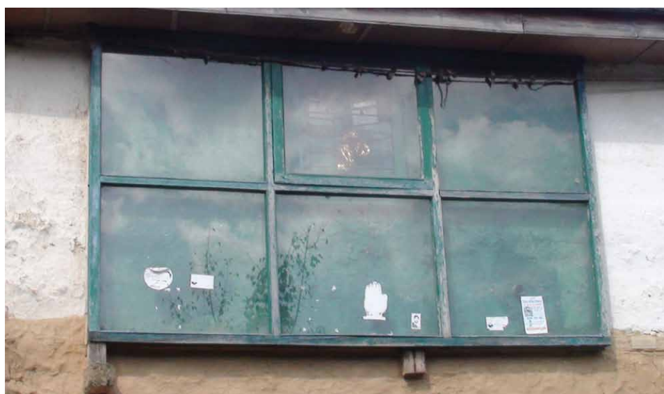
» Devaku's house with solar heating system (Trombe Wall type)
